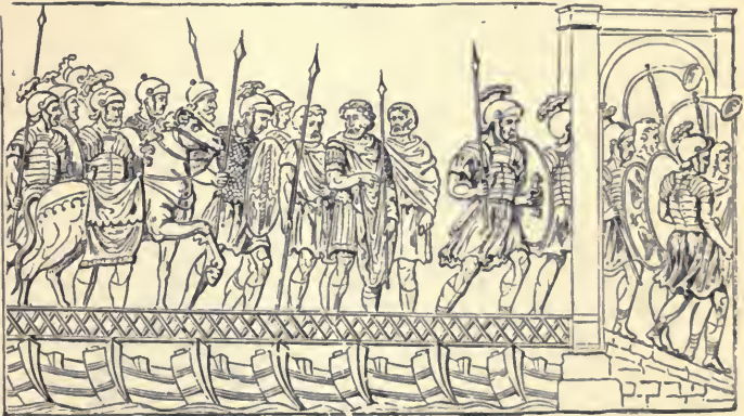
FIG. 55.—Bridge of boats.
